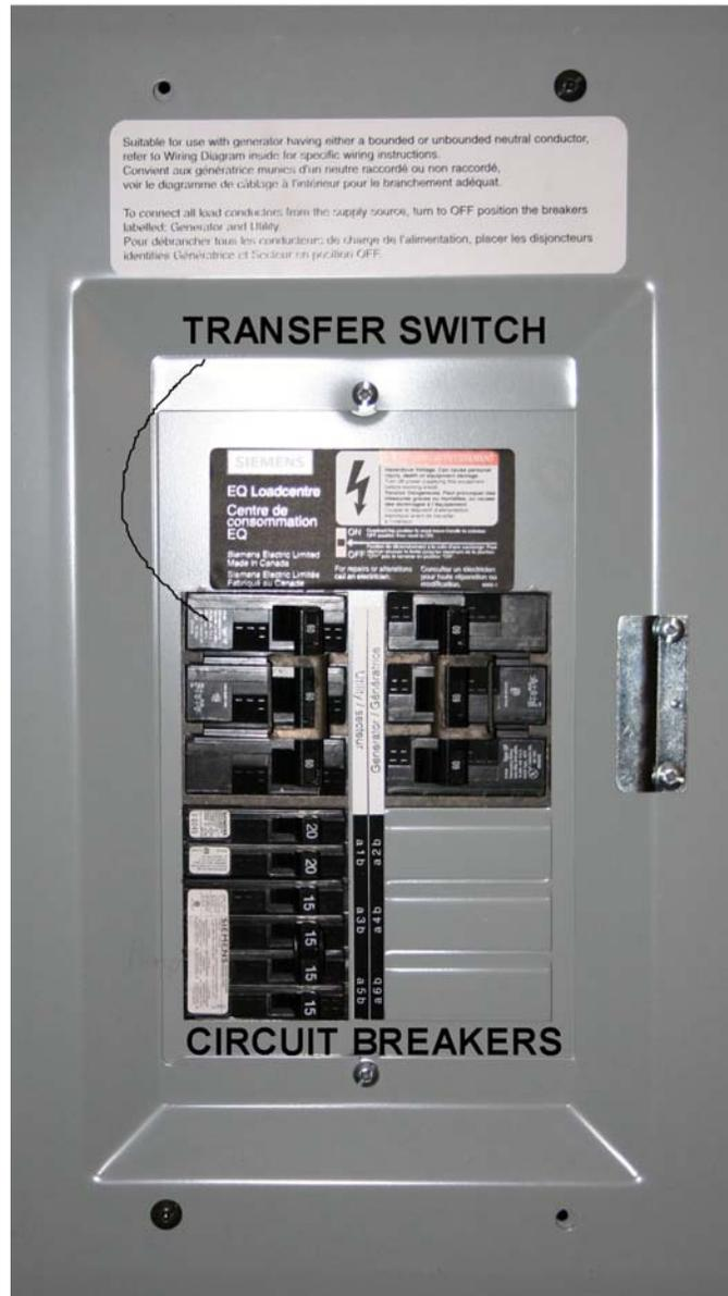
Shown above is the front panel of a Siemens generator panel (Catalog # EQG660D). See also, page 4 and page 15.
