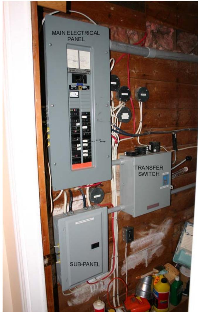
This is an example of a variation of the transfer switch type of installation. It is an older style using a separate transfer switch and sub-panel.
