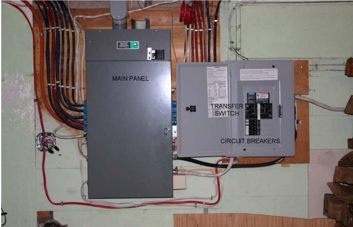
The system above uses a combination transfer switch and breaker panel as shown in the Transfer Switch method on page 4. This unit is manufactured by Siemens (Catalog # EQG660D).
