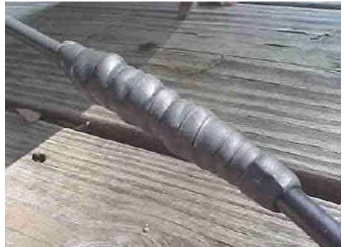
Figure 2 - The last wrap again comes straight back over the previous wrap without a diagonal. The seal is slightly sticky and should be molded now by hand to remove any gaps and to ensure that all the wraps are blending together. At some point the wraps will almost fuse together and the material may have to be cut away from the cable.
