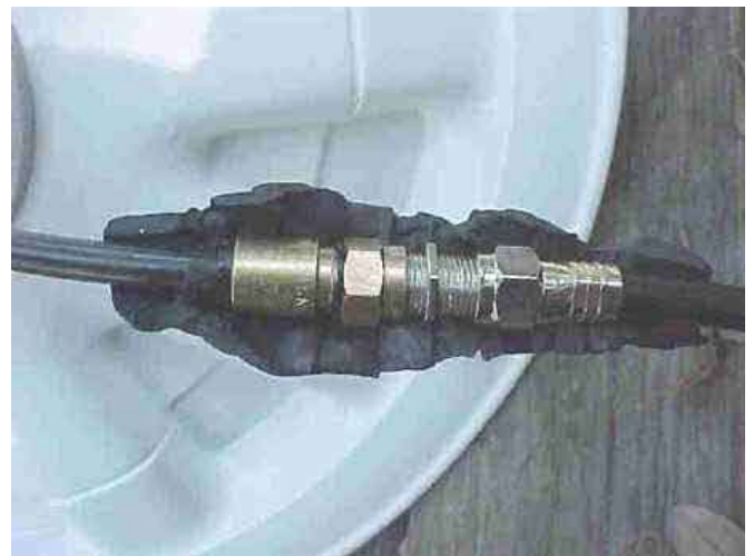
Figure 3 - View showing Coax-Seal cut away from the cable and connectors.
