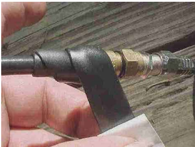
Figure 1 - Winding Coax-Seal tape. Note that the first wrap comes back on itself exactly, and the second turn starts the diagonal wrap. Wrap from the coax cover toward the fitting with one-half overlap with each winding.
