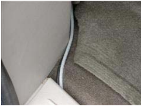
Figure 6 – Routing of the coaxial cable under the driver's side sliding door floor panel.
