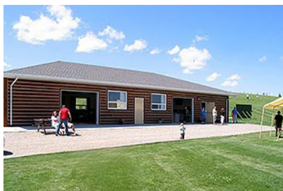
Exterior of the main building. Most of the meeting was held on the right half of the concrete slab while the meal was being prepared on the left side.
